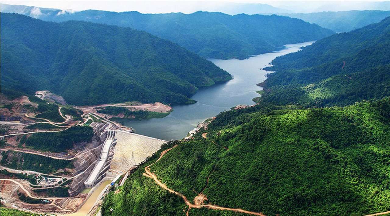
Nam Ngum 2 layout image below during construction:
